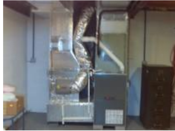
Heat pumps and basement air handler
