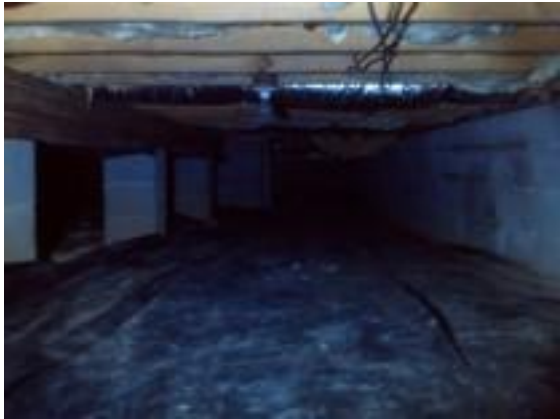
Vapor barrier is present in the crawl space.
