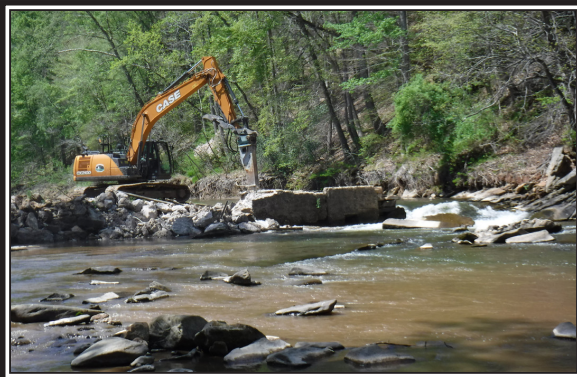
Drill and Broken Segments 4/25/2022
