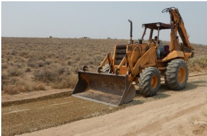
Below: Tribal maintenance worker spreading road base gravel.
