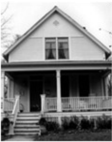
Farmhouse (Gable Front)
