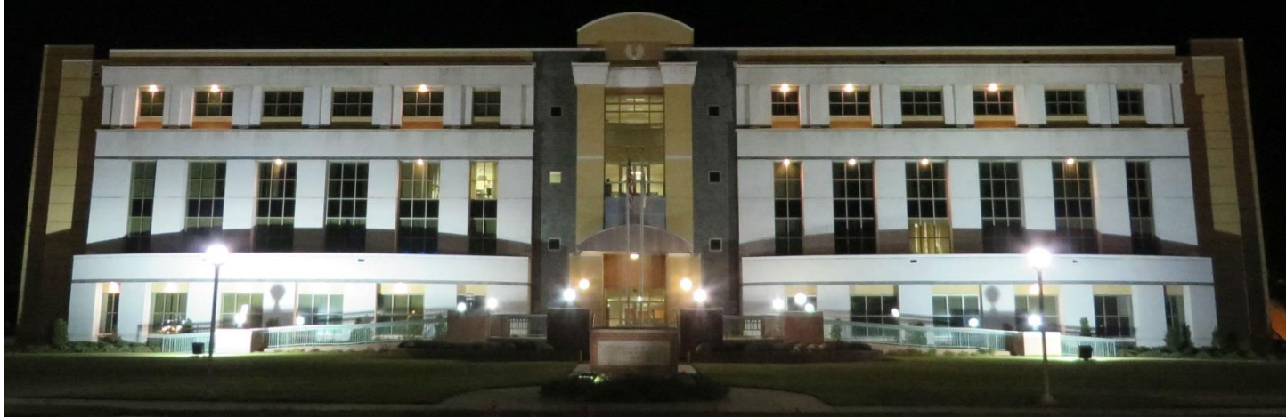
Sutton Administration Building
