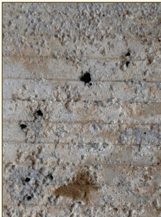
These photos show aluminum floors that are corroding and pitting from oxidation. These need to be repaired.
