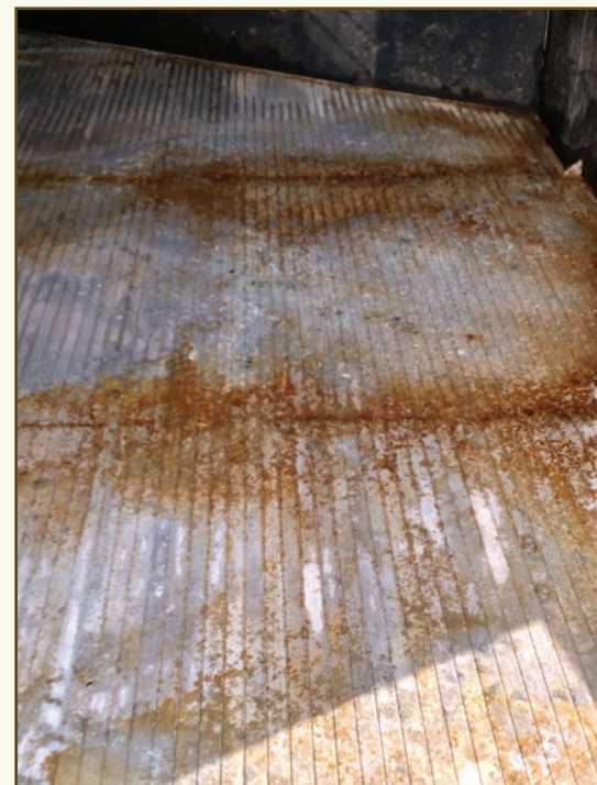
These photos show aluminum floors that are corroding and pitting from oxidation. These need to be repaired.
