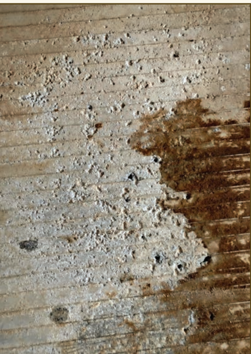
These photos show aluminum floors that are corroding and pitting from oxidation. These need to be repaired.
