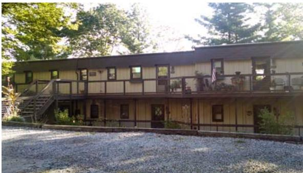
redesign of the existing mansard roof that went down to the deck, to accented shingles stopping at the top of windows and doors, which gives third floor owners an additional 2 usable feet of space on their front and back decks; repair of headers over sliding glass doors on the second floor and first floor, and on thresholds in the front and back, that needed replacing on the top floors; multiple coats of paint on entire building; new first floor back closets due to the original wood being
