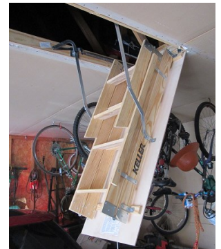
Partial extension of the attic ladder
