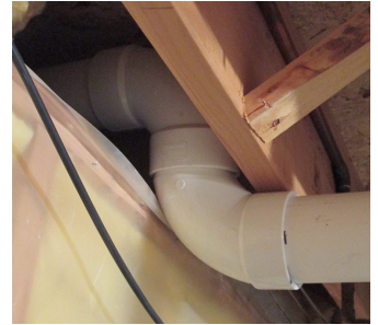
Elbow configuration to get up to the common garage joist.
