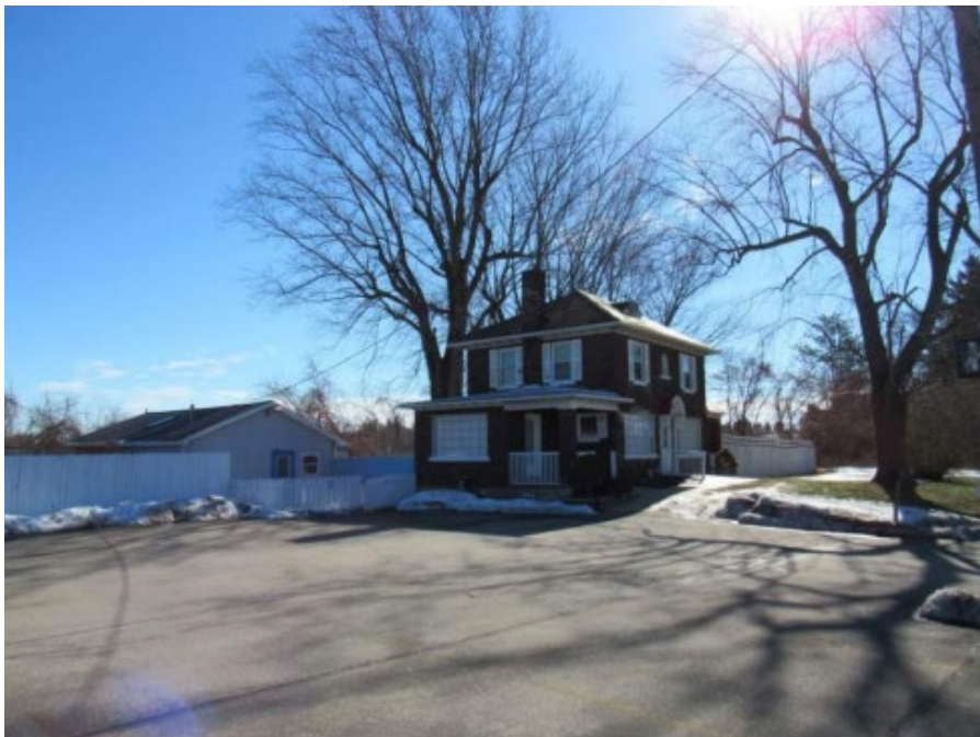
Photograph 2: North and west elevations of the Karl Weston House, facing southeast.
