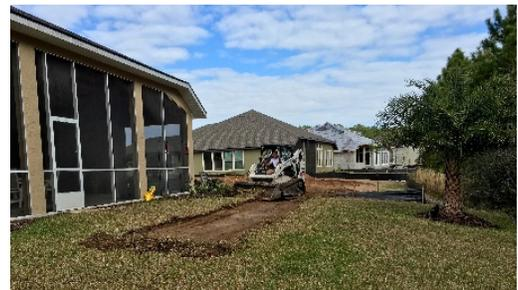
**Pool Layout:** This is the first step in the actual construction process. The excavation crew will set the form boards and your new pool will begin to take shape. Strict attention is given to critical dimension as our crew carves out the custom shape. Construction is typically 8 to 10 weeks from excavation.
