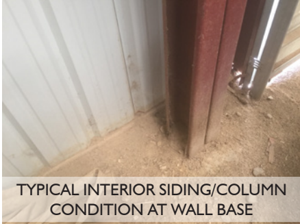
TYPICAL INTERIOR SIDING CONDITION AT WALL BASE
