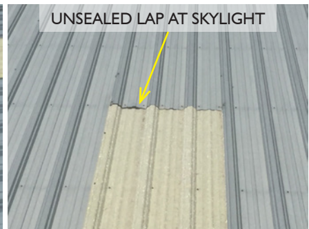
TYPICAL UNSEALED SKYLIGHT/ ROOF PANEL LAP
