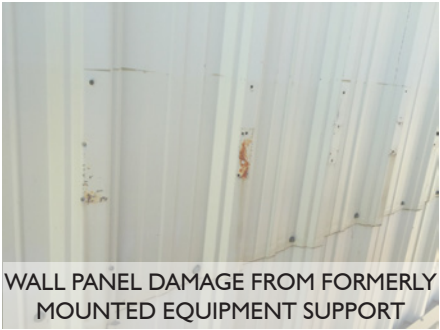
WALL PANEL DAMAGE FROM FORMERLY MOUNTED EQUIPMENT SUPPORT
