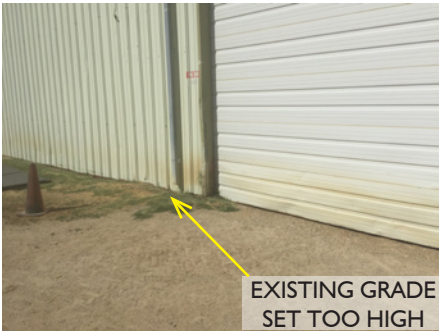
DAMAGED/POORLY MAINTAINED WALL PANELS
