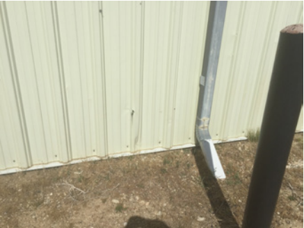
DAMAGED SIDING AT OVERHEAD DOOR
