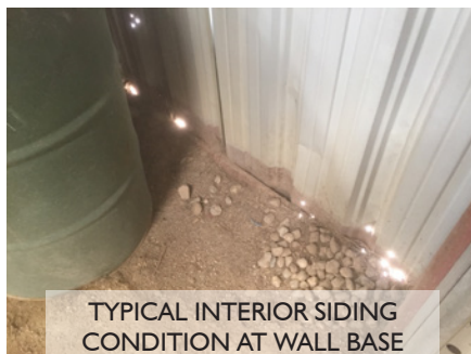
CONCRETE SLAB POURED AGAINST METAL SIDING - INTERIOR CONDITION
