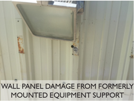
WALL PANEL DAMAGE FROM FORMERLY MOUNTED EQUIPMENT SUPPORT
