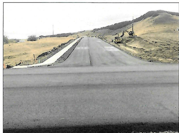
W 2nd Street uphill to new cul-de-sac
