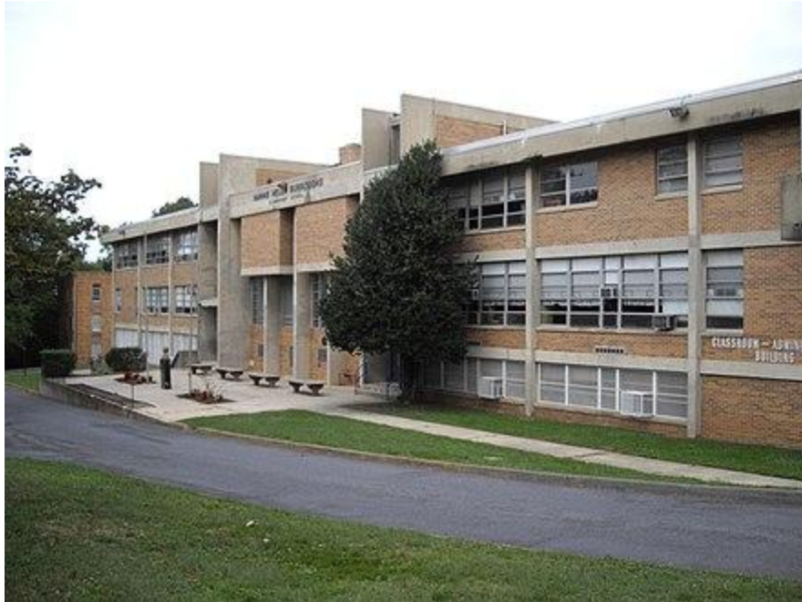
Nannie Helen Burroughs’s Trades Hall sits at the southeast corner of 50th Street NE and Nannie Helen Burroughs Avenue NE. 4
