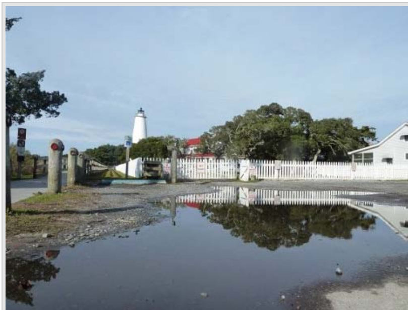
Standing water near the lighthouse over a week after a rain.
