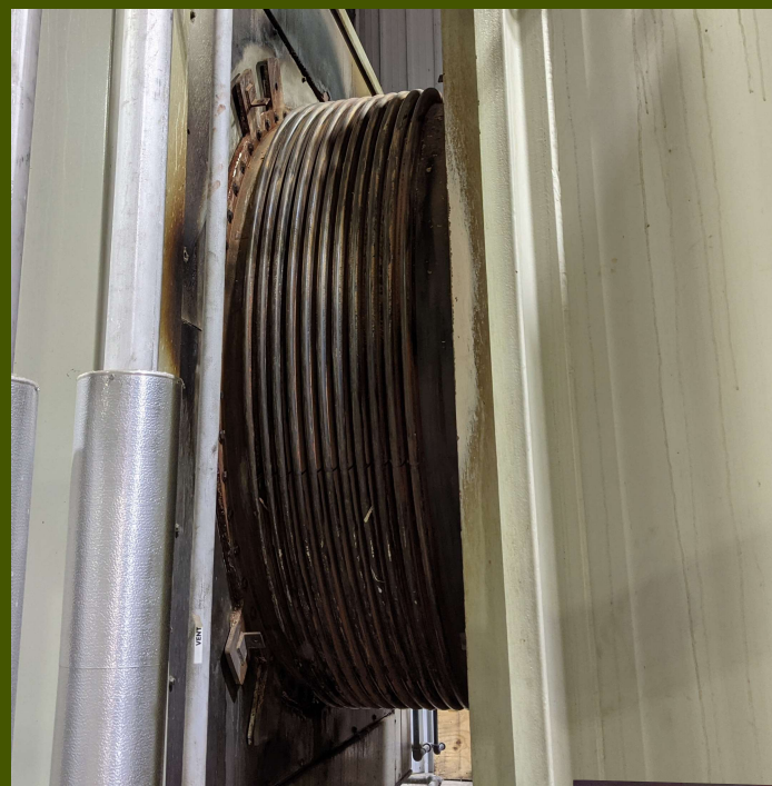
Leaking Bellows to Floating Liner and Expansion Joint Belt System
