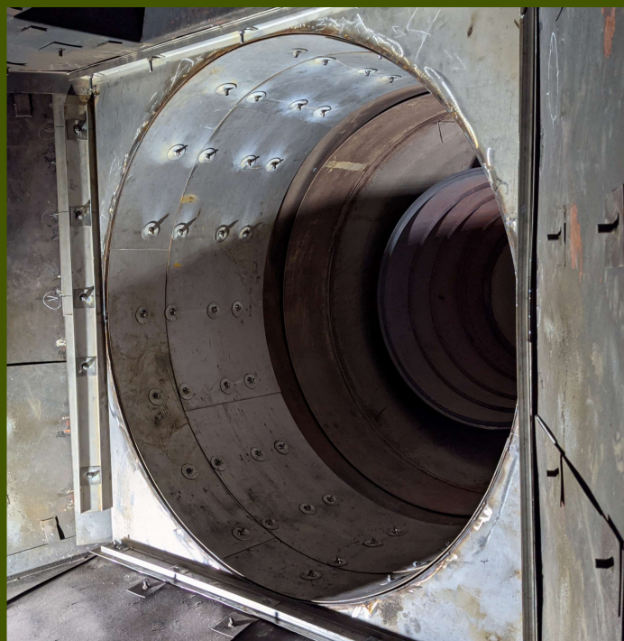
Internal Liner System Instead of Bellows Flow Shield - Same Gas Path, Increased Wall Thickness
