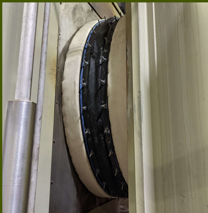
Leaking Bellows to Floating Liner and Expansion Joint Belt System
