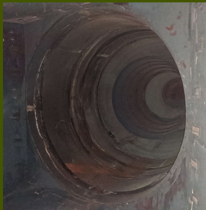
Internal Liner System Instead of Bellows Flow Shield - Same Gas Path, Increased Wall Thickness
