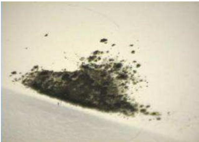
**Advanced case of ceiling mold infestation** growing on, inside, and probably also above the ceiling itself [hidden mold growth].
