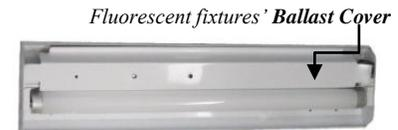
Figure 2 - Fluorescent Tube Fixture with Diffuser Removed
