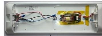
Figure 7 - Fluorescent Tube Fixture Showing (+) & (-) Wires, as well as Switch (if unit is so equipped)
