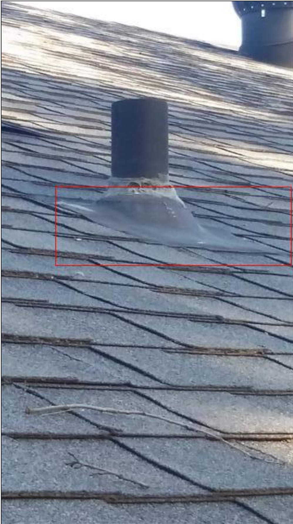
1.1 Item 1(Picture) plumbing vent on back of home
