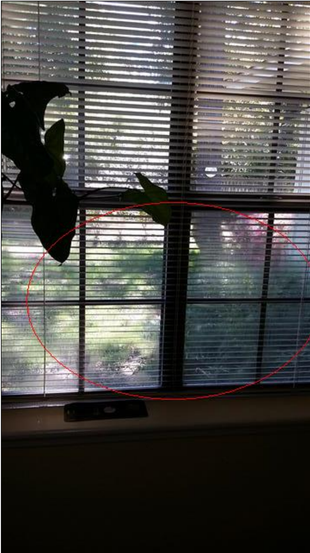
2.2 Item 1(Picture) windows in dining area of kitchen
