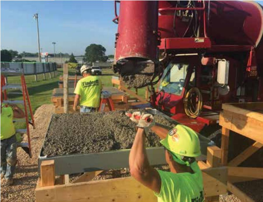
Photo 3: Exterior concrete slabs being poured at SRI Consultants' facility in July 2016
