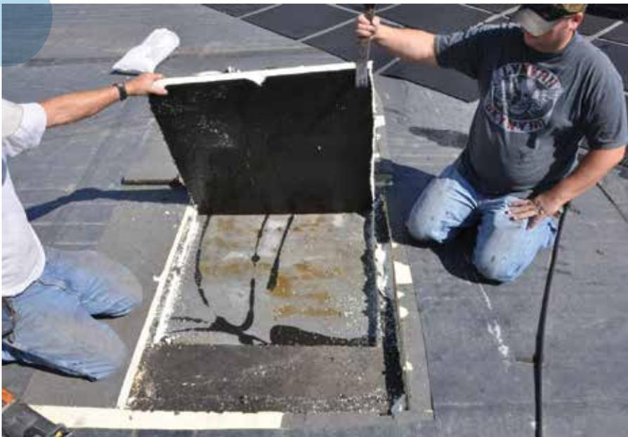
Photo 1: This roof system was installed over a lightweight structural concrete deck in the upper Midwest. The roof had only been in place for a matter of months before wind delaminated the moisture-weakened polyisocyanurate facer at the membrane level. Small amounts of condensed moisture are visible on the concrete surface.
