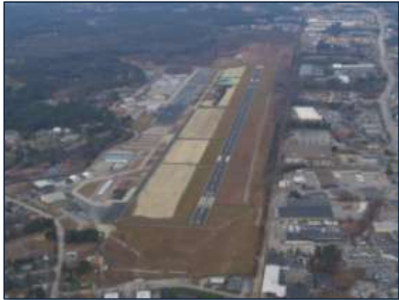
New runway construction at Nashua Municipal Airport (Boire Field)
