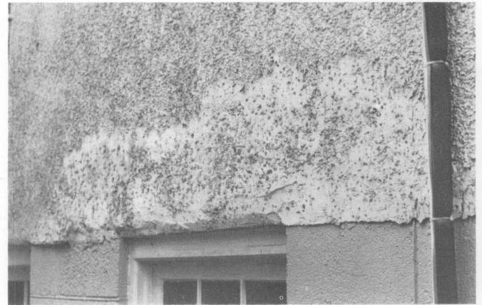
Fig. 14. This poorly executed patch is not the work of a professional plasterer. While it may serve to keep out water, it does not match the original surface, and is not an appropriate repair for historic stucco. Photo: Betsy Chittenden.
