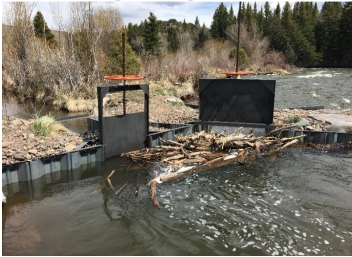
River headgate looking downstream
