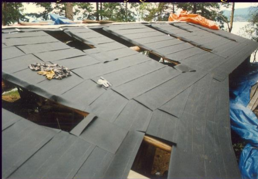
North Roof w/30lb. Felt And Skylights Looking West
