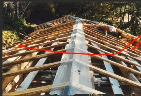
Installed Rfaters Note The 2 X 4 Spine On Walls
