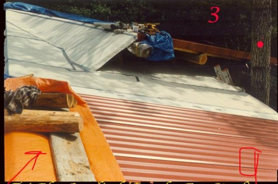
Tri Ply Applied (Ready For Steel)
