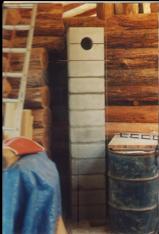
Second Pipe Hole Above And 90 Degrees From Previous
