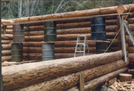
East Wall Two Windows To Be Cut Later
