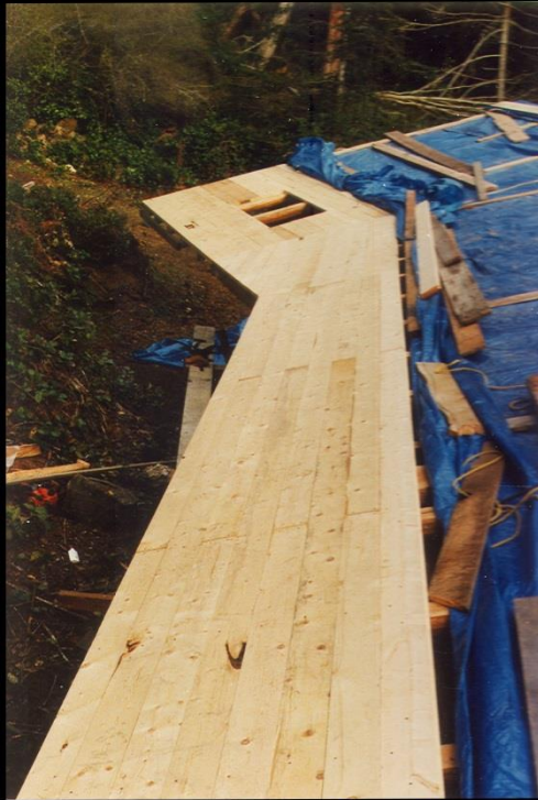
Beginning North Roof Looking East
