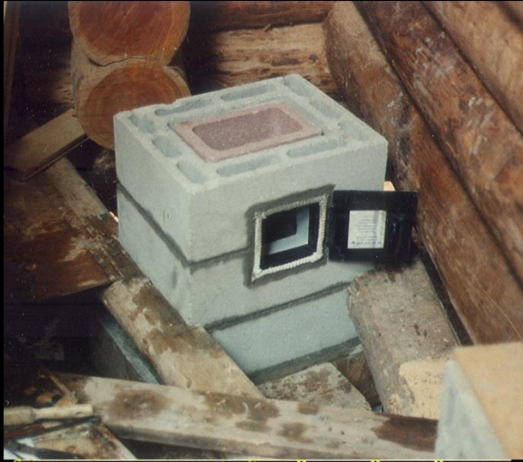
Chimney. Material 17" x 21" x 8" Cement Block. With *8" x 12" x 12" Pumice Liner. Chimney Base Is A Poured Cement Block Resting On A Conglomerate Matrix. Two Floor Joists Were Notched To Allow Construction Through Floor
