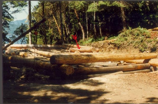
Hefty Log (with red arrow) In Place
