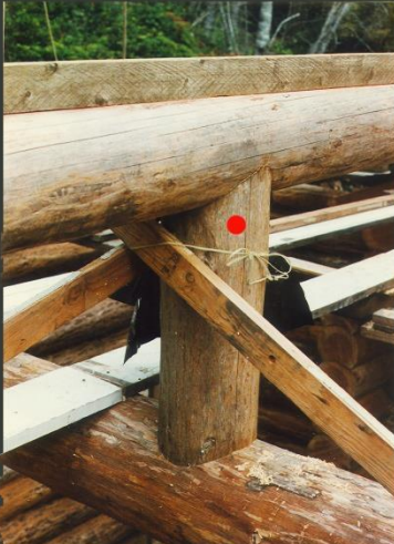
Middle Of West Ridge Pole Setting On West Crossbeam
