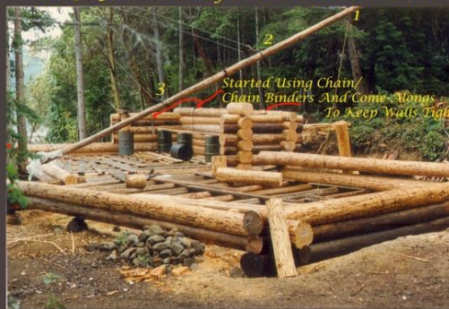
Note: The Gin Pole Boom Now Has Three Blocks
