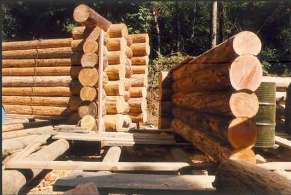
Back Door Bathroom Wall Looking North
