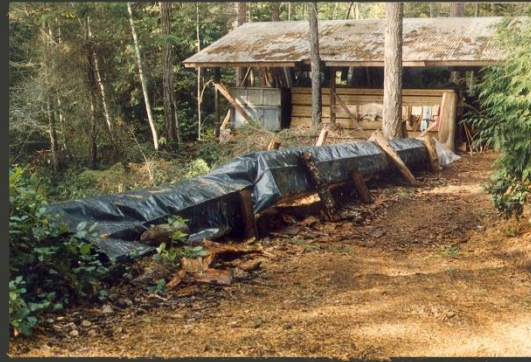
Covering Logs For Winter 10 mil Polyethylene
