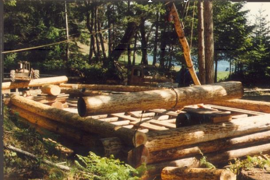
Maneuvering First West Window Log
