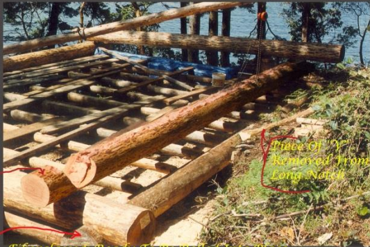
Fiberglassed, Ready To Be Rolled Into Place Note: The rear end of the log does not have any material removed (rare) because the log beneath was not as long.
