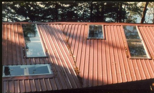
North Roof Finished With Valley and Skylights Facing South
