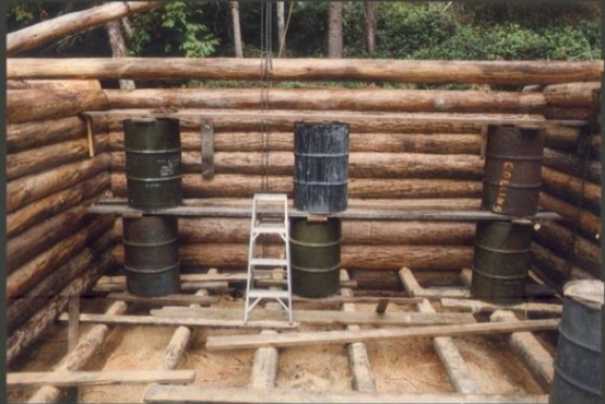
Scaffolding In Bathroom
