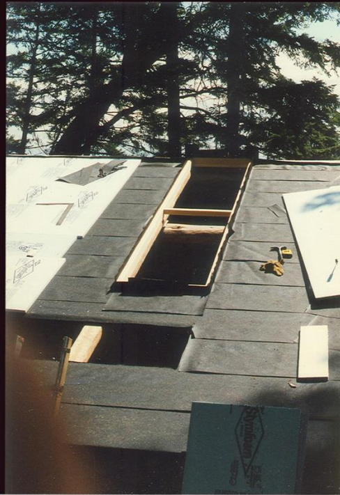
North Roof Facing South Ready For styrofoam
