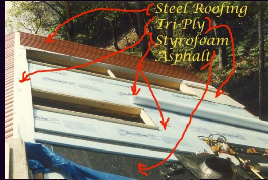
North Roof Looking West
