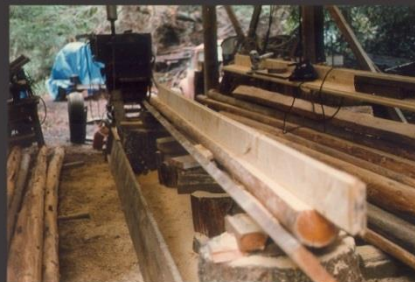
Checking Flatness Of Milled Rafter
