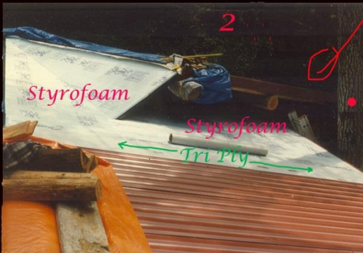
Styrofoam, Tri-Ply and Steel Applied Over 30 lb Felt To Southwest Section
