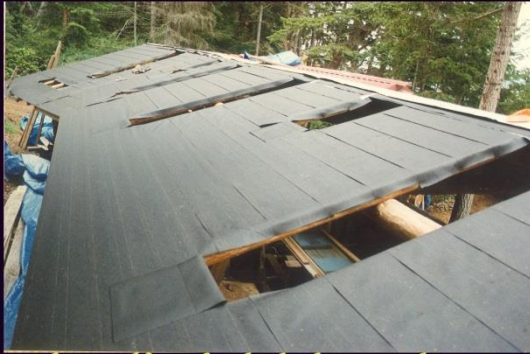
North Roof With Skylights, Looking East
