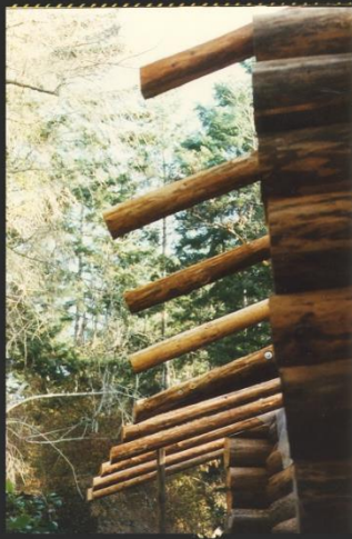
Porch Rafters North Side
