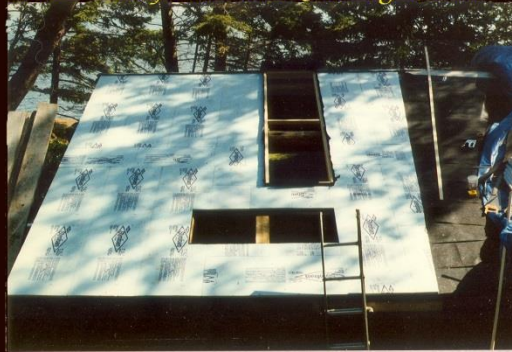
North Roof Facing South w/Styrofoam and 30 lb Felt
