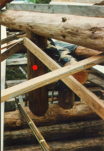
West End Of East Ridge Pole Setting On Kitchen Wall Partition
