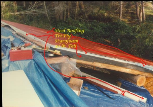
Southeast Roof Nearing Completion
