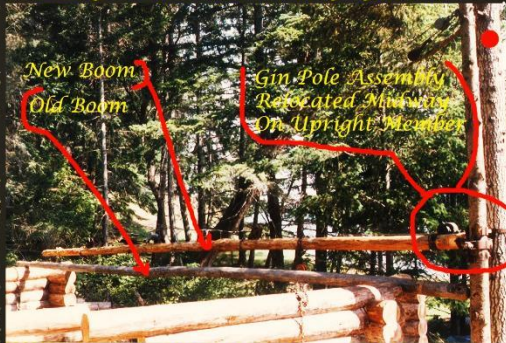
New Gin Pole Assembly Installed
