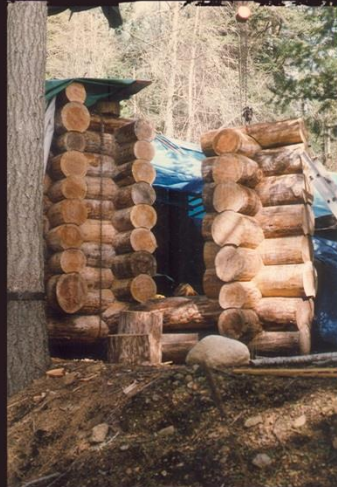
Outside Looking East
