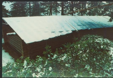
Winter Cover Supported By Rafters
