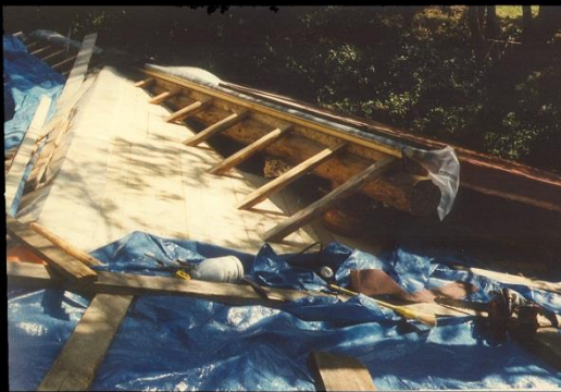
Valley Rafters Between The Two Sections Of the South Facing Rooves
