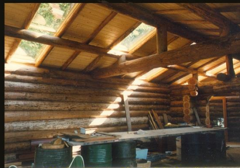
Northwest Interior After Skylights Installed Facing East
