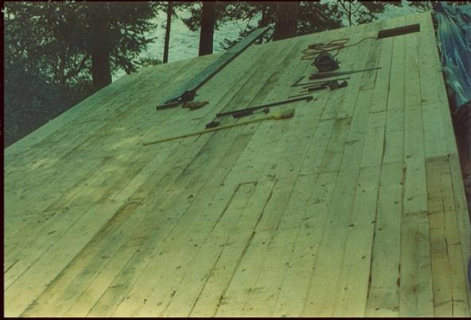
Southeast Roof (w/ chimney Hole) Looking West
