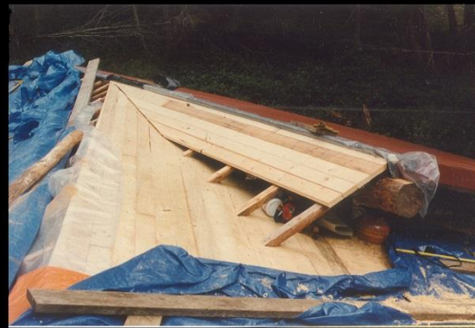
Nailing SPF Roofing To Valley Rafters
