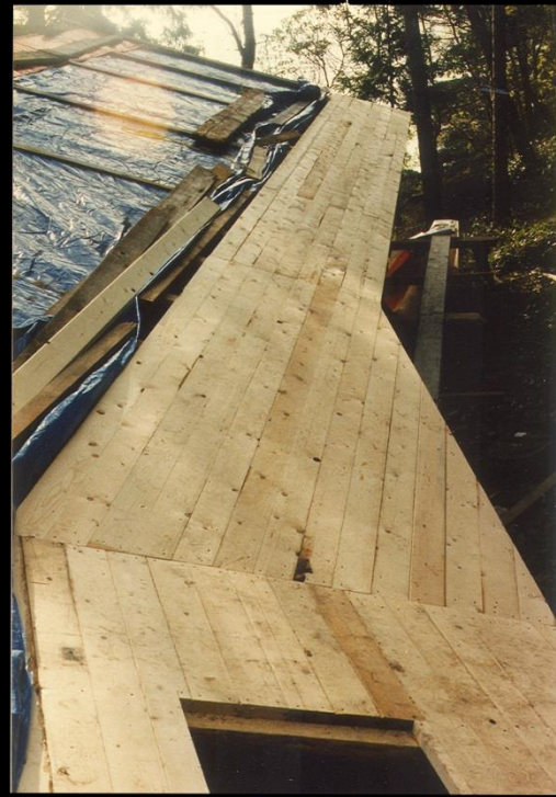
Beginning North Roof Looking West
