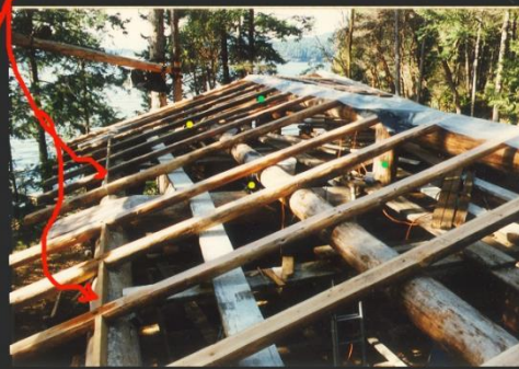
Installed Rfaters Note The 2 X 4 Spine On Walls
