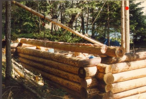
The 36 Footer Ready To be Rolled Into Place
