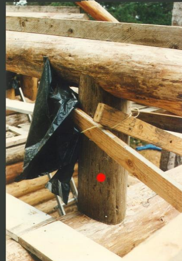
Middle Of West Ridge Pole Setting On West Crossbeam
