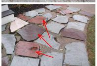
3. General overview of exterior. Exterior Surface Exterior steps/stoop/landing. (Not attached to Deck or Porch.) NOTE: LOOSE TREADS due for correction.
