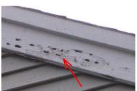
6. General overview of exterior. Exterior Surface Corner boards NOTE: Sections of DAMAGED corner boards due for correction.
