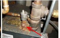
29. CELLAR Heating System Flue Pipe METAL ~ NOTE: RUST on flue pipe due for correction, contact plumber for corrections now.
