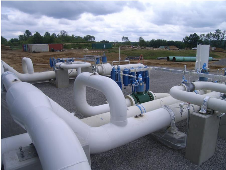
**Figure 2 Regulation and Measurement Station**
