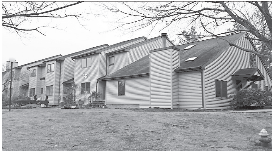
Reina Renovations recently completed the work on the 82-unit, 14 building Deep Run Townhouse development on Route 9 in Old Bridge.
