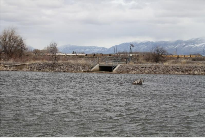
Headgate (from diversion dam)
