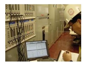
TDS can install and utilize specialized, temporary vibration instrumentation equipment to fully instrument a machine that has no permanent vibration monitoring equipment.
