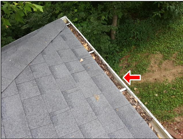
2.4 Item 6(Picture) front right corner of home
