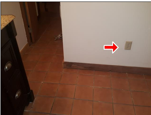
7.6 Item 3(Picture) basement bathroom
