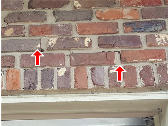
3.0 Item 1(Picture) right side of garage
