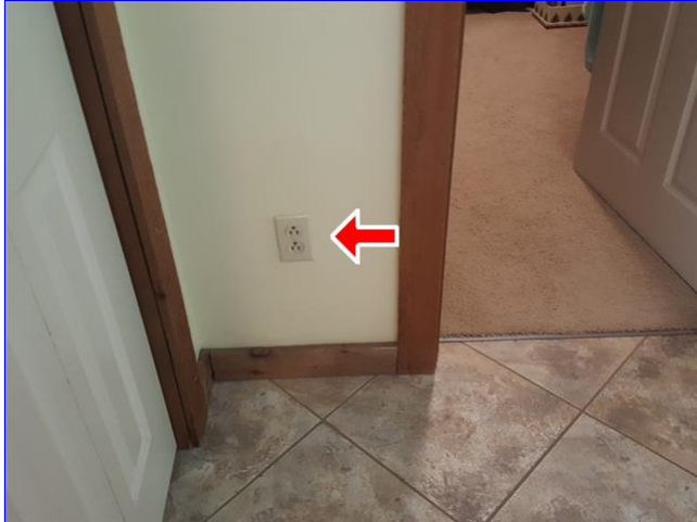
7.6 Item 1(Picture) master bathroom
