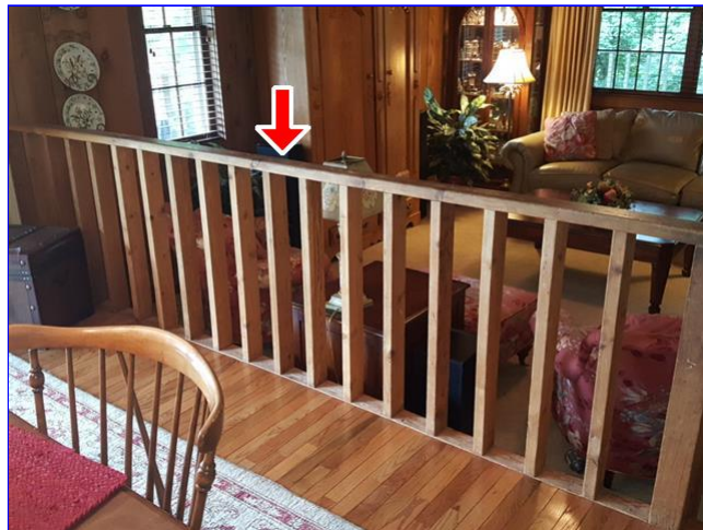
6.3 Item 1(Picture) dining room
