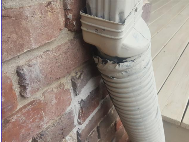
2.4 Item 3(Picture) front center of home
