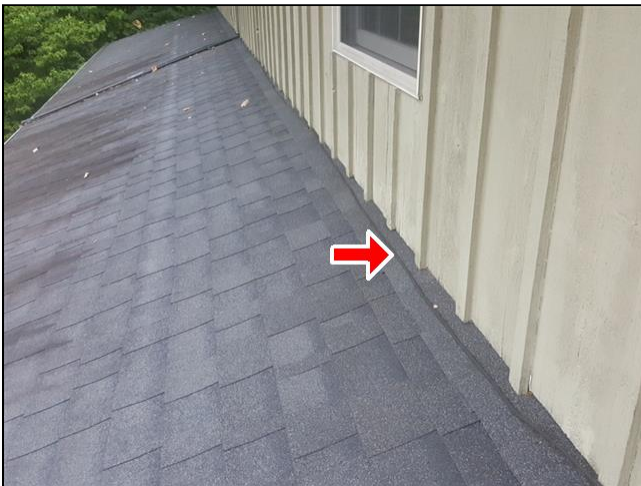
2.1 Item 3(Picture) rear of home
