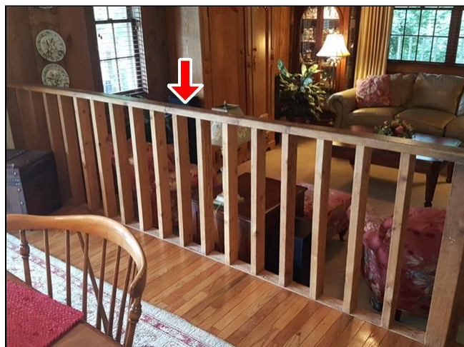
6.3 Item 1(Picture) dining room
