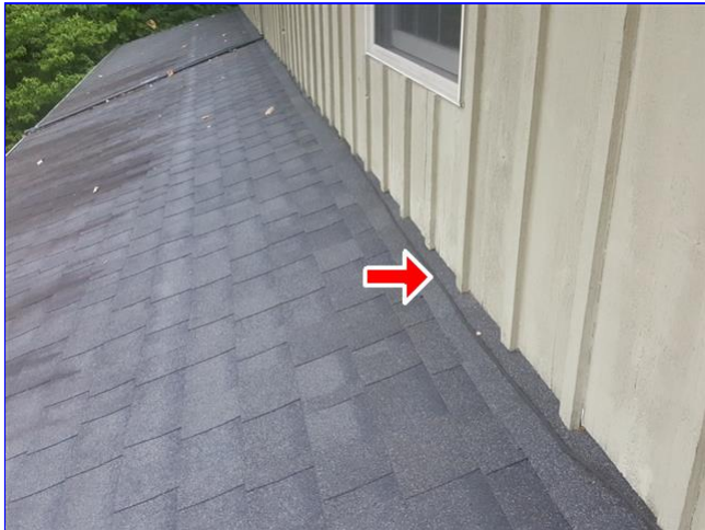
2.1 Item 3(Picture) rear of home
