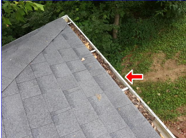
2.4 Item 6(Picture) front right corner of home
