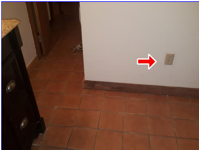
7.6 Item 3(Picture) basement bathroom
