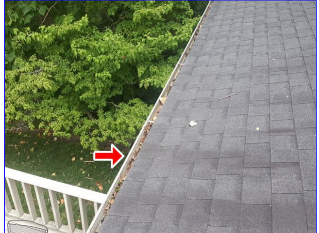
2.4 Item 7(Picture) rear left side of home
