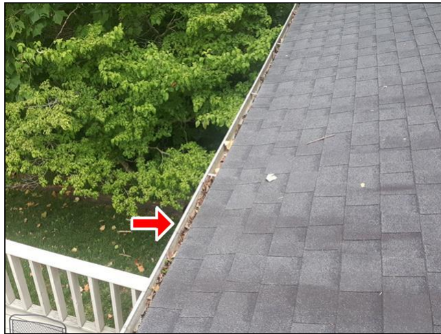
2.4 Item 7(Picture) rear left side of home
