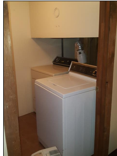
basement washer dryer room
