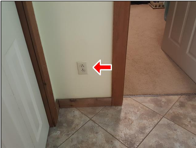
7.6 Item 1(Picture) master bathroom
