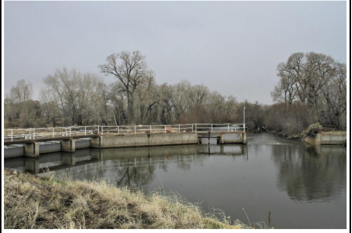
Headgate and diversion dam
