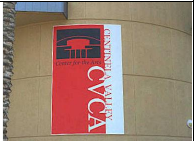
TS23- Printed vinyl stretched on the curved frame
