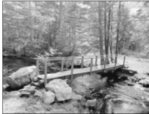
The bridge over Collins Brook in the Miller Family Forest.
