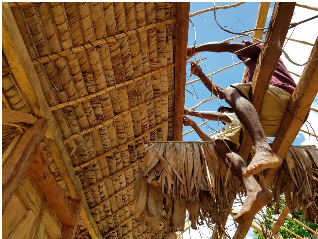
◀ A beneficiary ties his roof onto the frame, taking on the required beneficiary participation
