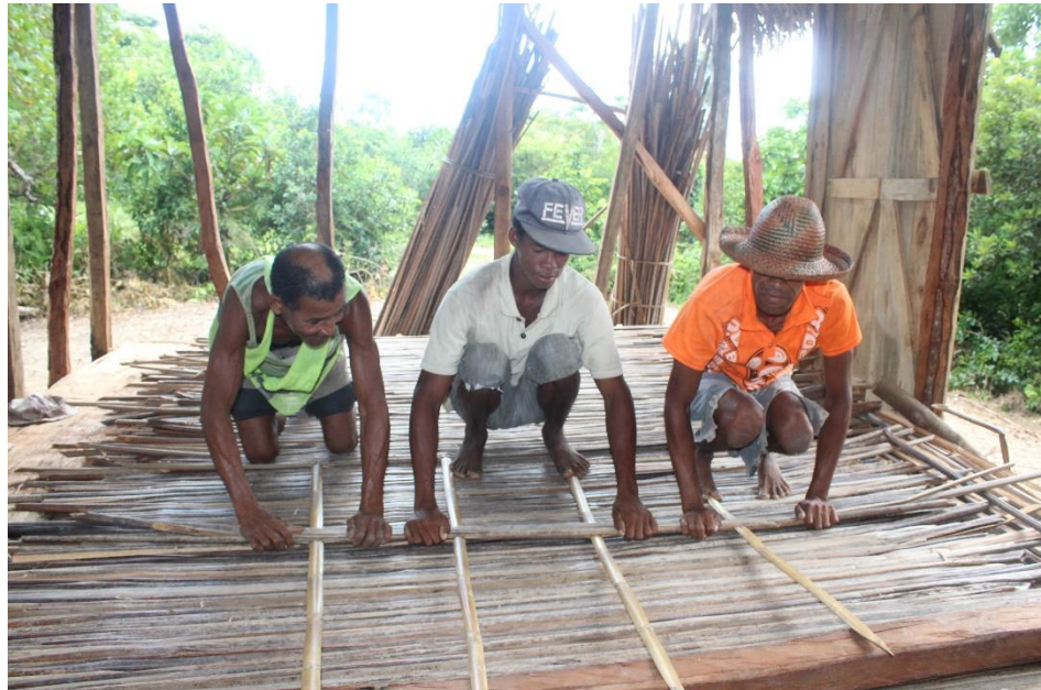
◀ A beneficiary ties his roof onto the frame, taking on the required beneficiary participation
