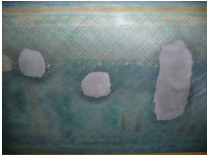
Fig. 12. Previous repairs become visible after blasting with Type VIII – no damage!
