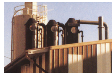
Tri-NO x scrubber through-the-roof installation.
