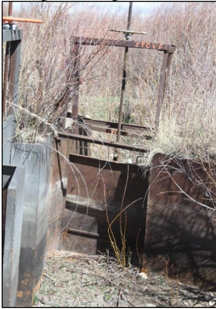
Headgate looking downstream
