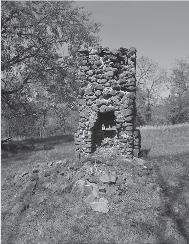
Chimney No. 4. This chimney was cleaned of overgrowth but did not need restoration. Note the method of creating the lintel. Photo courtesy of Bernice Walker.
