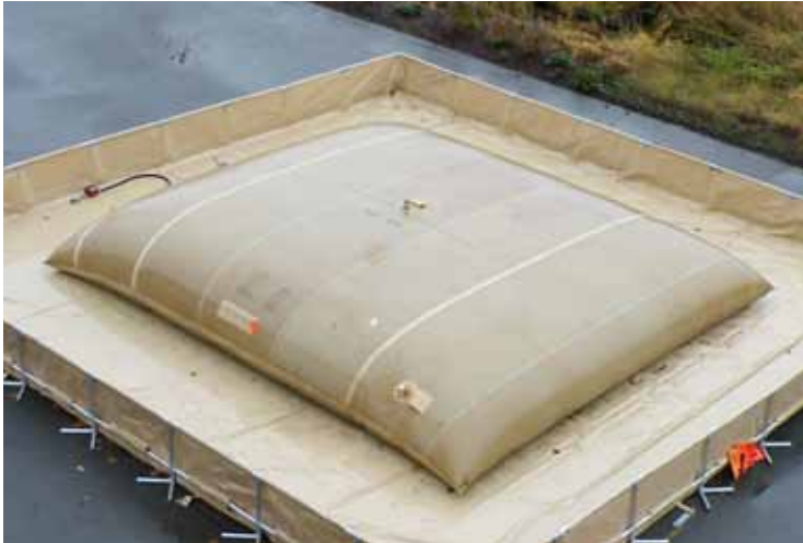
Terra Tank inside an Insta-Berm (Frame).
