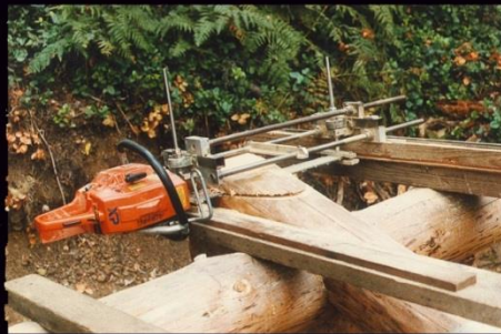
Shaping The Wall Timbers And Cross Beams To Conform To The Roof Line Set At The Width Of A 2 x 4 On End (Above The Top Wall Log)
