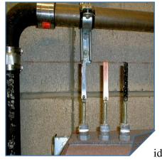
**How They Work.** Corrosion coupons are pre-weighted, and usually rectangular strips of metal that are of the same metal make up as your system's components. The corrosion coupons are typically installed in a corrosion coupon rack and exposed to system conditions for a determined amount of time.
