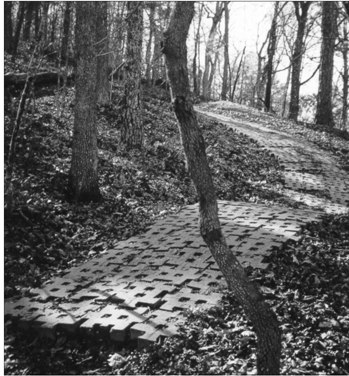
This picture shows the conlock blocks in use on trail 130A
