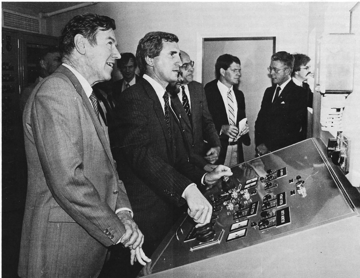
Mr Brereton operates the control console which activates the fire fighting system at the Bulk Liquids Berth at Port Botany during its commissioning on 18 June last. The former president of the MSB, Mr John Wallace, is pictured in the foreground. On Mr Brereton's left, partially obscured, is Mr Rick Foster, engineering manager (NSW) for Wormald's Fire Systems, designers and installers of the fire control apparatus. On Mr Foster's immediate left is Mr Eric Silva, Port Manager, Sydney Ports.
