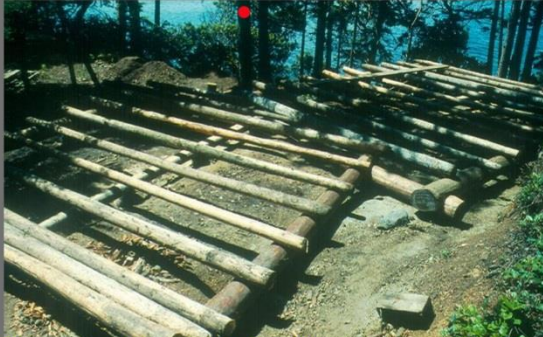
Floorjoist Layout w/#1 thru #7 Logs In Place
