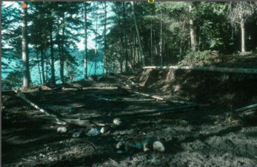
Laying Out Cleared Site
