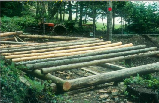
Laying Out Of Floor Joists
