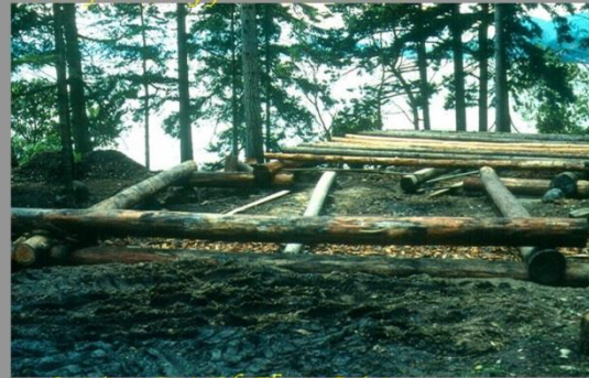
Laying Out Of Floor Joists
