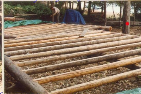
Finishing Off The Last Few Joists
