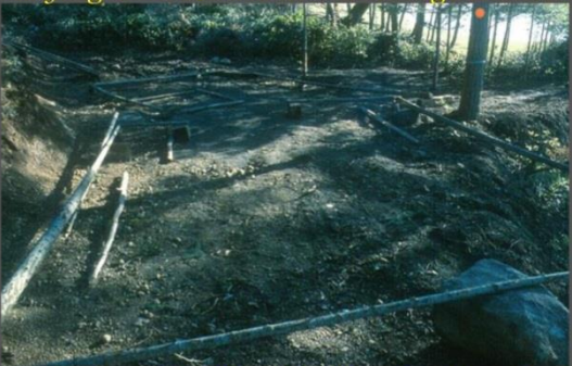
Laying Out Site Looking Southeast
