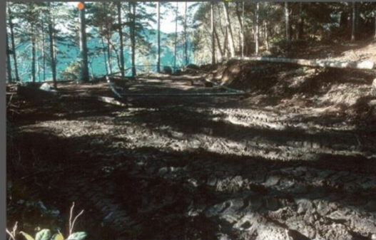
Cleared Site Looking W Start Of Layout
