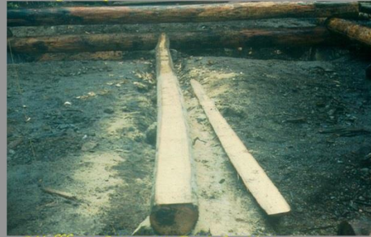
Midfloor Support East Section
