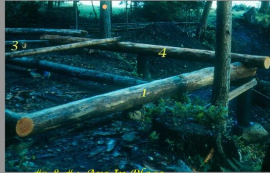
#3 & #4 Are In Place
