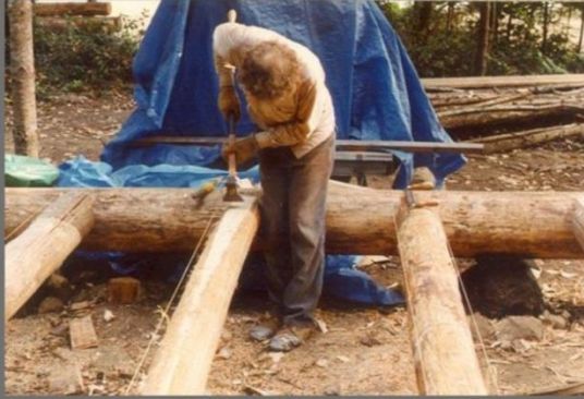
Working The Chalk Lines (In Pairs)
