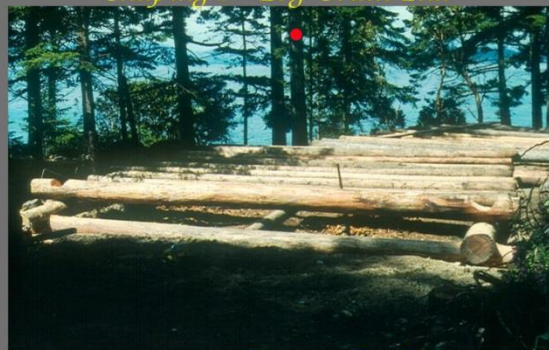
# 8 Log Ready For The PV
