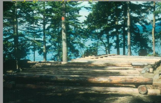
Laying Out Of Floor Joists
