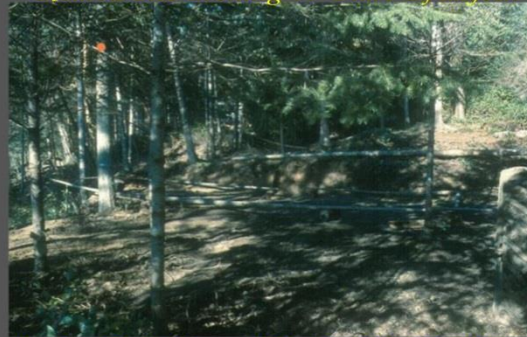
Laying Out Cleared Site Looking Northwest
