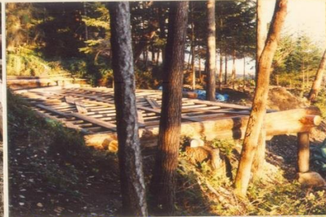
Most Of The Floor Joists Leveled
