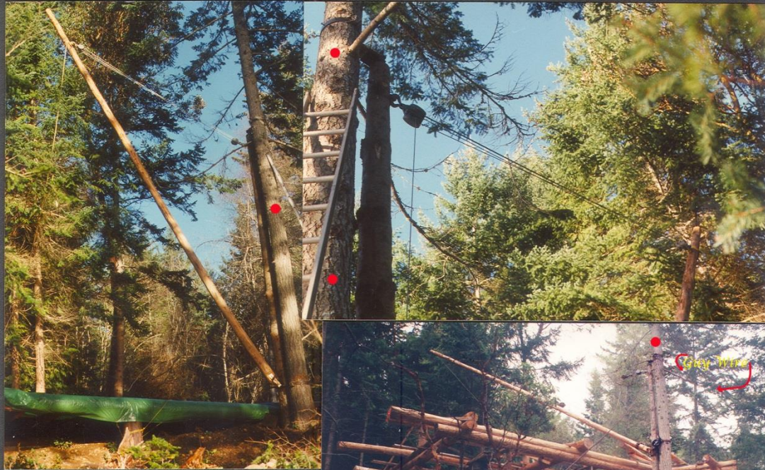
First Configuration Of Gin Pole
