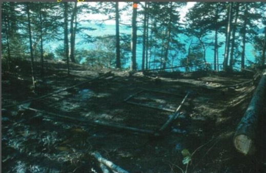
Laying Out Cleared Site Looking Southwest
