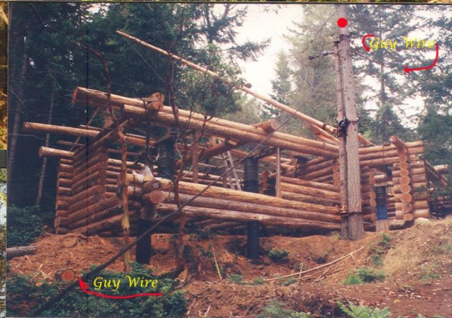
First Configuration Of Gin Pole
