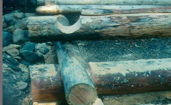
Shaping # * Log South End
