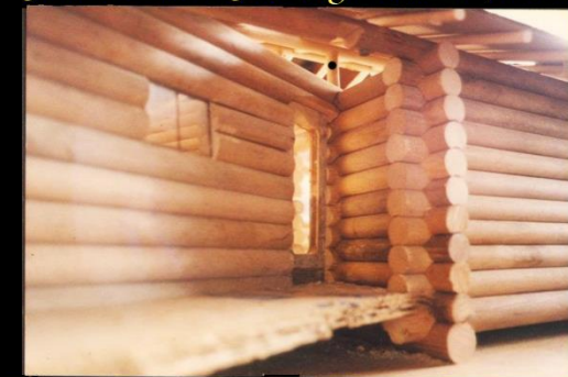
Rear Door Covered Porch (North)
