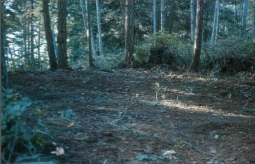
Clearing Site Looking West
