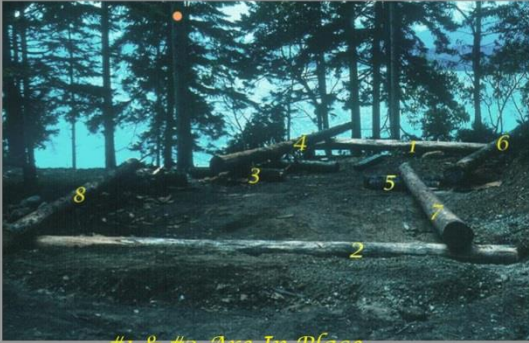
#1 & #2 Are In Place
