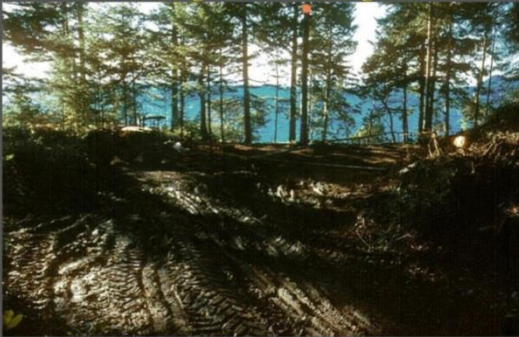
Cleared Site Looking Southwest
