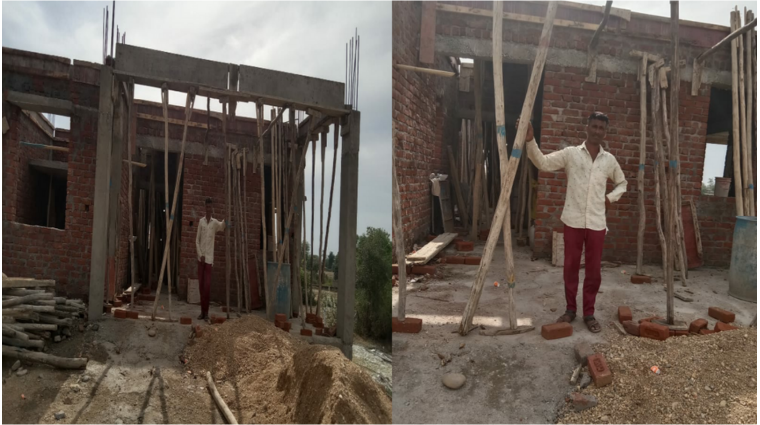
Poonji Lal building a roof
