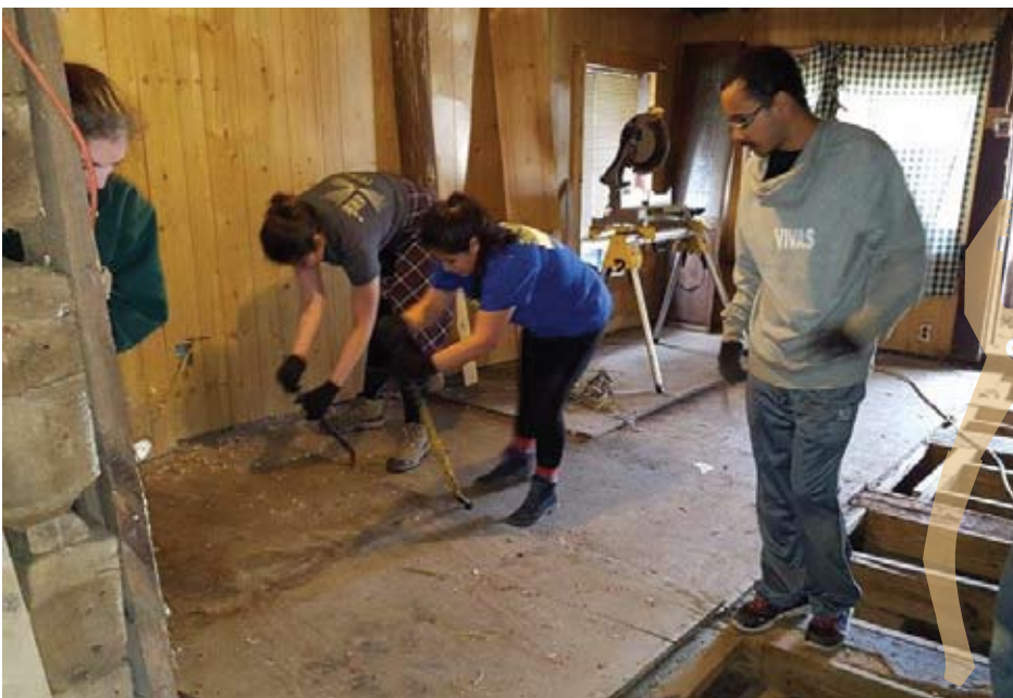
Volunteers working on the home renovation project in War, WV-2016
