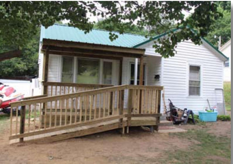
A home after rehab completed in Cleveland, TN-2016
