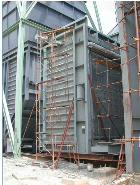
Conversion of simple cycle elbow to fully functional diverter for an Alstom GT13E2 in Viet Nam
