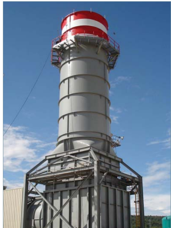
Convertible simple cycle exhaust stack in Venezuela
