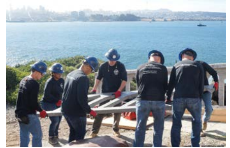
Transporting 300-pound precast concrete panel up hill
