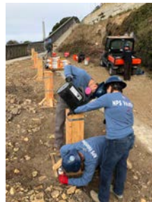
Constructing walkway at base of stairs
