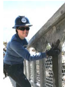
Installing welded wire mesh for visitor safety
