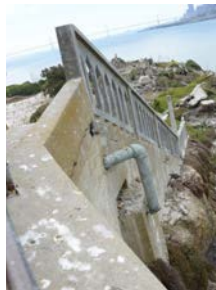
Completed stair railing from cliff side
