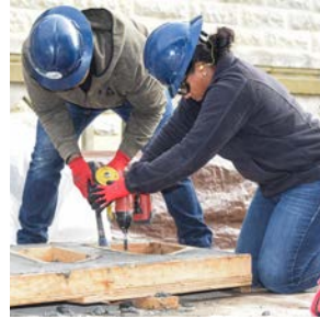
Removing formwork from completed precast panel
