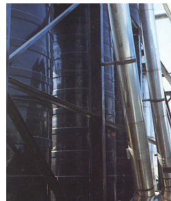
Gas transfer duct between stages
