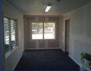
We worked on the porch of the Hobby House and replaced and rebuilt all of the old termite damage and drywalled the entire porch.
