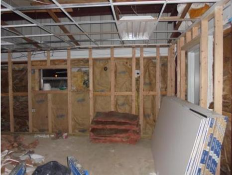
Completely tore apart Paul Rife room and remodeled. new walls ,insulation, drywall ,floor, ceiling, bathroom and A/C.
