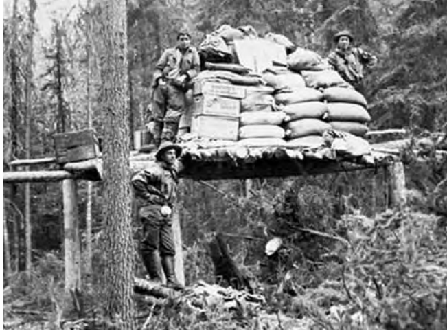
Figure 6—Surveyors supply cache on the 21st baseline near the Athabasca River (Alberta). Library and Archives Canada / PA-020500 . 1913
